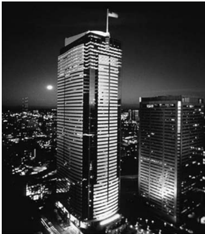
Figure 9.4 Two Union Square, Seattle. Courtesy of Portland Cement Association.
