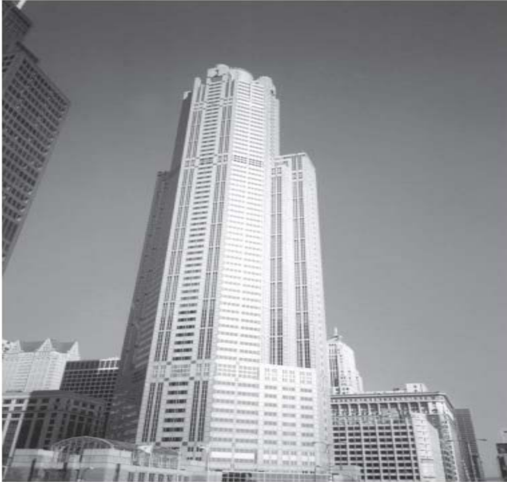
Figure 9.1 311 South Wacker Drive, Chicago – high strength concrete used in columns.
